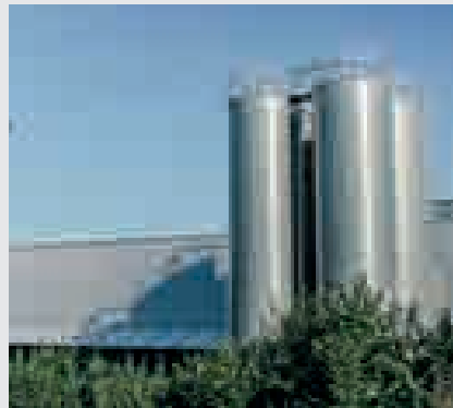
■ Silos for raw materials
