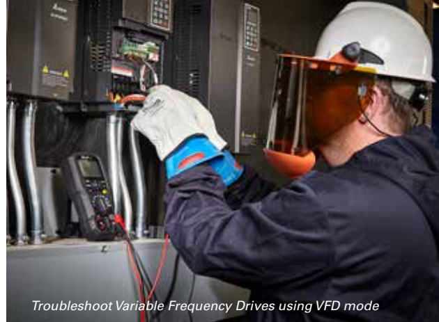
Check if voltage is present with the built-in Non-Contact Voltage detector (NCV)
