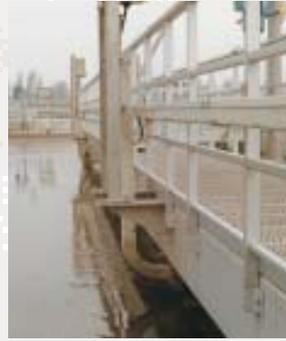
Energy Distribution water and recycling, power stations, nuclear plants, extraction and mining, gas...
