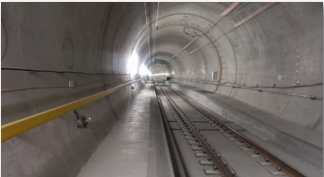
Gotthard Base Tunnel, Switzerland
