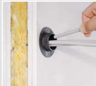
Insert the new cables.
