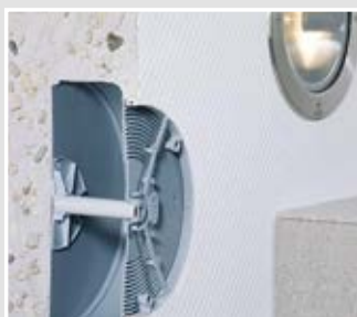
Pre-mount the housing with the installation kit.
