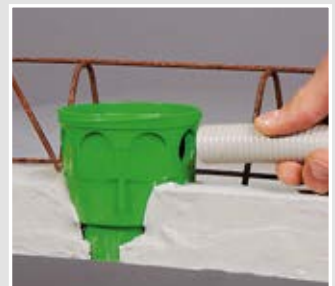
The conduit is inserted tightly and accurately and the box is sealed with the cover.
