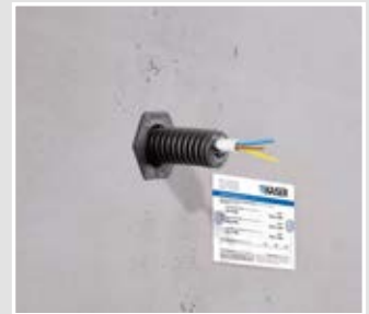
Wall feed-through in concrete fire-protection wall.
