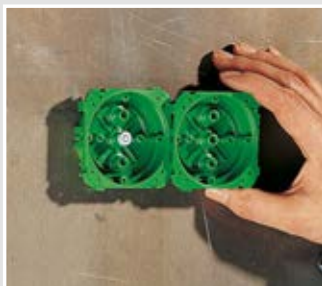
Attach front part to formwork.
