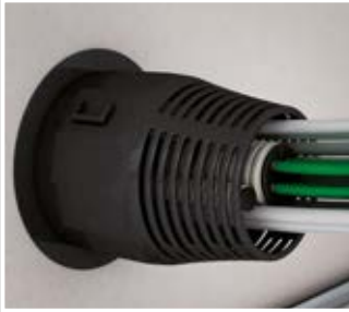
Mixed population of sheathed cables and conduits.
