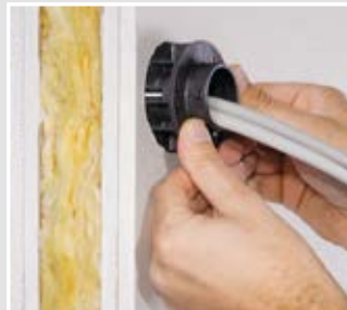
Press the sealing cylinder into the installation opening.
