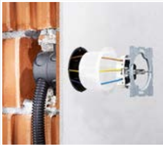
Later air-tight closing of flush-mounting boxes.
