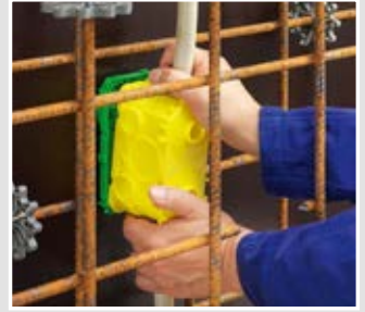
The snap-in connection ensures fast installation.
