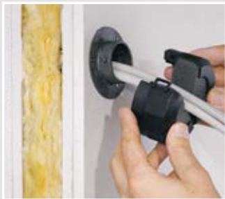
Place the sealing element around the cables and close it.
