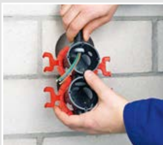
Creating installation opening.
