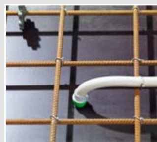
The surrounding conduit lock retains the conduit securely in the holder and ensures the correct function of the empty conduit system
