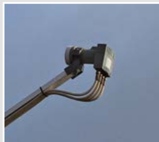
4 coaxial cables are connected here for reception.
