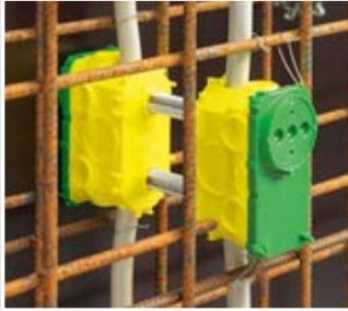
Opposing installation, cable entry behind the reinforcement.
