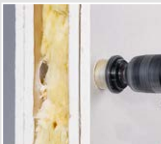
Cut a 35 mm installation opening using e.g. a KAISER Multi 4000 cutter (1082-10).
