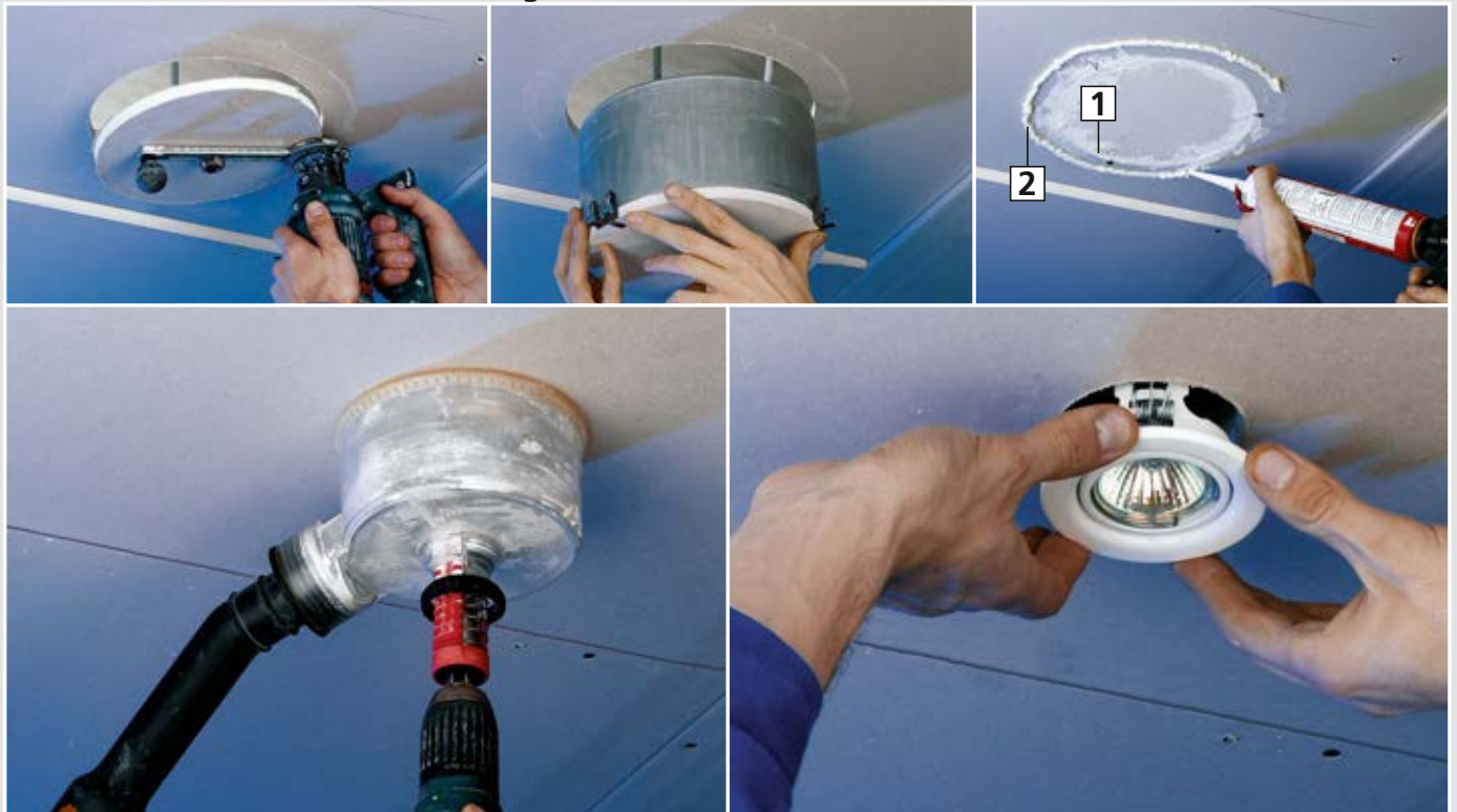
1 Edge joint | 2 Sealing bead
