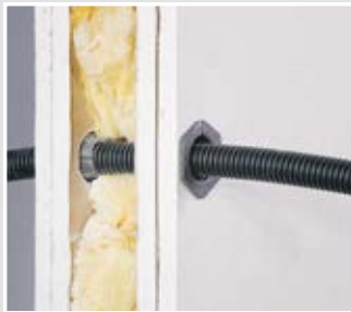
Wall feed-through in plaster-board fire-protection wall.
