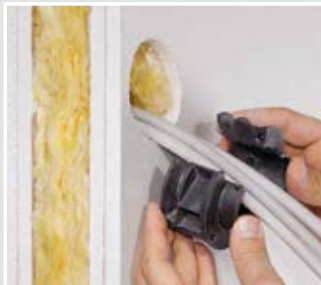
Place the two-part sealing cylinder around the cables and press together.
