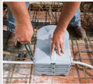
Also secure the housing to the reinforcement.
