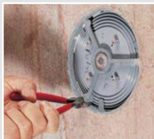
After removing the formwork: remove the bridges and open the front part.
