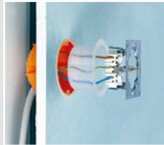
Later air-tight closing of cavity wall boxes.
