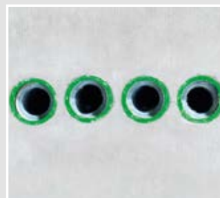
After striking the formwork, there is only a minimal visible area in the concrete.
