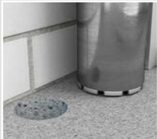
Making a core drill hole 150 mm or 100 mm.
